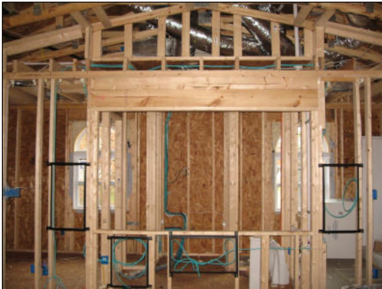
built. US Nippura used typical 2x4 construction with doubled 2x8s as headers. You're A/V integrator will be able to make sure the framing coincides with all speaker, wiring, and cable requirements.
