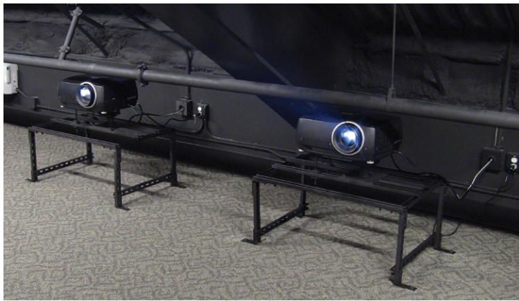
Two projectors feed the auditorium's 84"x212" rear-projection screen.
