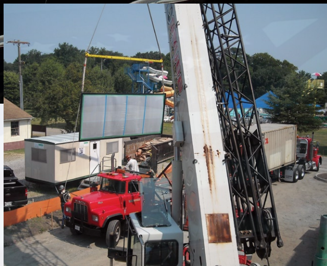
The second-floor, 210-seat, 50'x50' auditorium features a 84"x212" rear-projection screen. The 1200-pound screen presented installation challenges, requiring the efforts of 13 men to move it into position.
